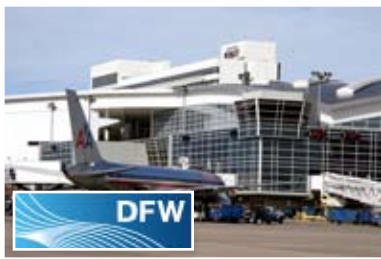
DFW Airport Terminal D
